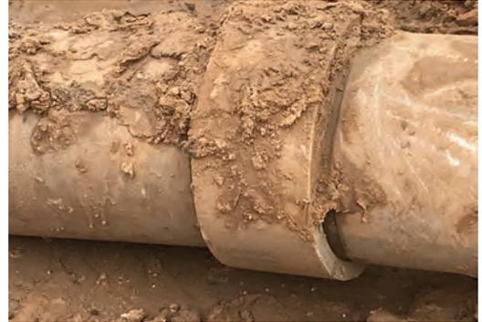
The A/C coupling was removed along with a section of A/C pipe. The JCM 204 Reducing Coupling (customer built length) was installed on the A/C pipe and the substitution HDPE pipe was installed on the other side.
