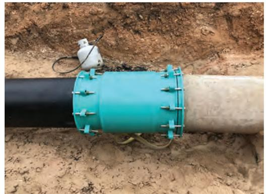
To reinforce the connection and ensure the pipe did not pull out from the coupling under pressure, fabricated restraint systems were provided for both the HDPE Side (JCM 610) and the Asbestos Cement Side (JCM 630).
