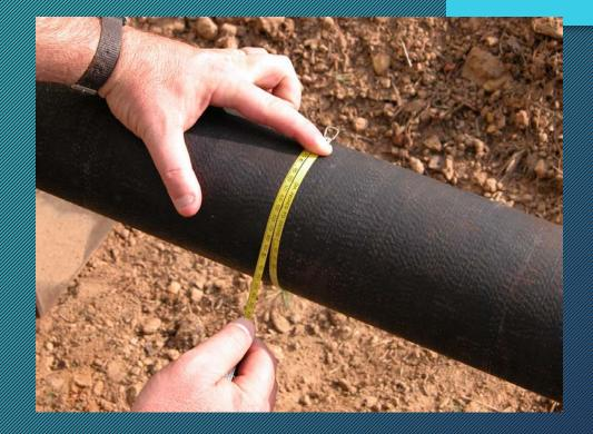
After measuring the pipe, confirm the size and range printed on the box label and...
