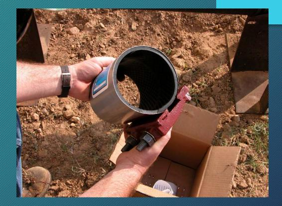
Loosen the nuts (do not completely remove); swing the bolt free from the open ear finger lug.
