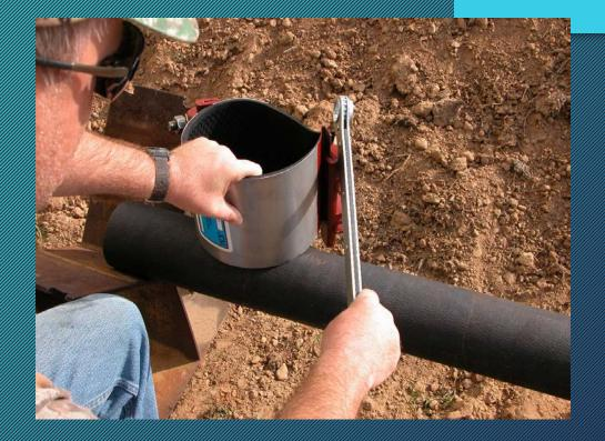
When the lug has been removed, set it aside in a clean, safe place free from dirt, sand or debris that could impede reinstallation of the lug.
