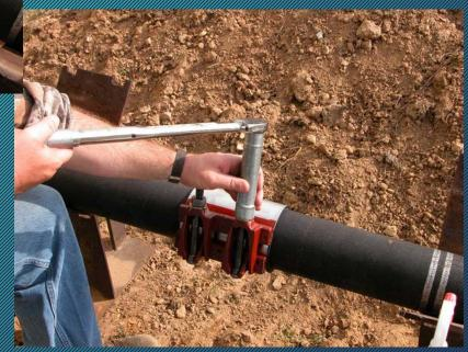
For the 171 Removable Lug is the Open Ear Lug. Note the Open Slots for the oval neck bolts. This is the lug section that is removable.
