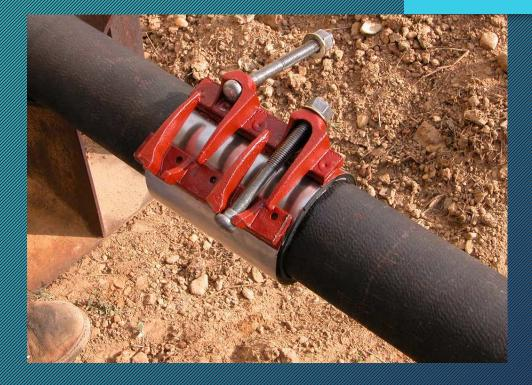
Rotate clamp in direction of the arrow to ensure gasket is laying flat – crimps and folds will create a leak channel and the repair will fail (eventually).
