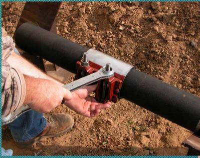
Confirm proper torque levels with torque wrench.
