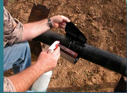
When clamp is installed around the pipe, reinstall the open ear lug onto the stainless receiver band. Again, if necessary, gently tap the lug with a hammer or wrench to start it back onto the band.
