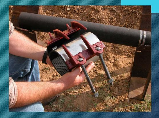
Lubricate the pipe surface with water or soapy water mixture. Do not use a oil base pipe lubricant. The oil creates a film between the gasket and the pipe preventing a water tight seal.
