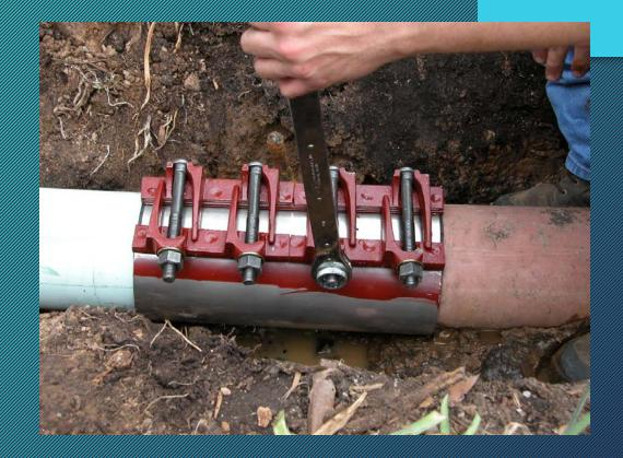
Before installing the clamp, review installation instructions. Instructions include the step by step procedure to pipe preparation, clamp installation and bolt torque requirements.
