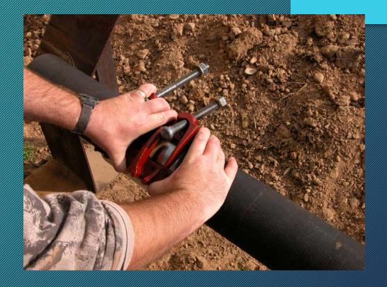
Mesh fingers and engage bolts into open ear lugs. Do not tighten bolts.
