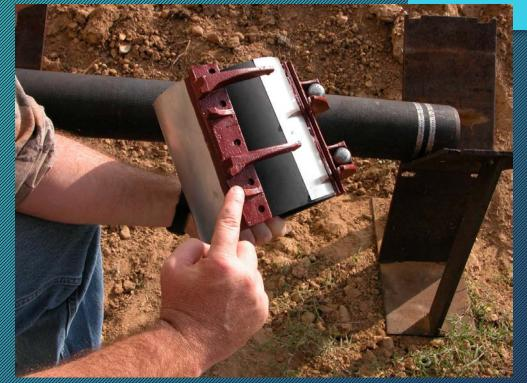
If necessary, lug end may be tapped with hammer or wrench to loosen and assist removal.
