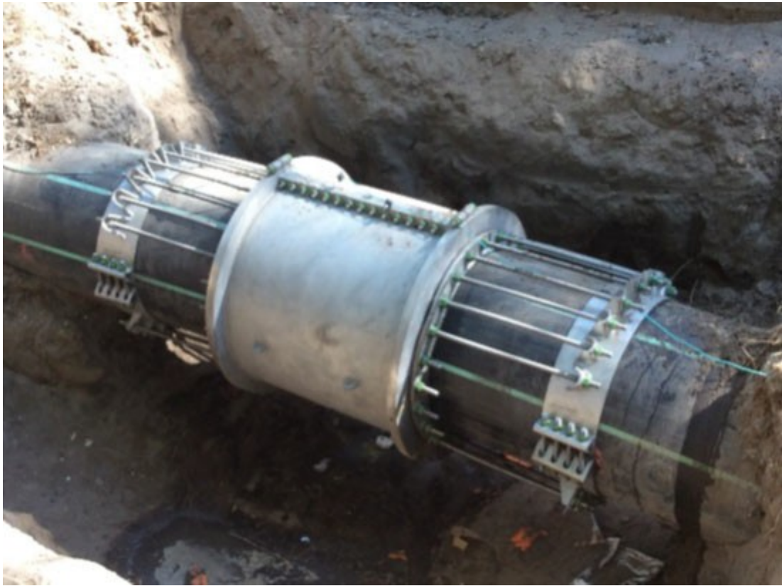
Figure 1. Encapsulation can be an attractive, cost-saving option in complex applications where disruption to the service is highly problematic or where the mechanical complexity of conventional repair approaches makes them simply too labor-intensive or expensive.
