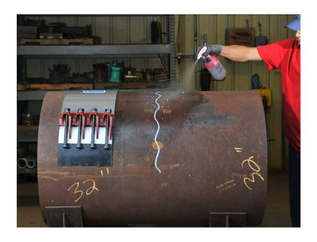
Spray or pour soapy water around the damaged area to lubricate the pipe to make installation of clamp easier. Soapy water provides a slippery surface to let the gasket slide on the pipe into place and is water-soluble. Do Not Use Oil Base Pipe Lubricant – it does not break down with water and will not allow the gasket to adhere to the pipe for water tight seal.
