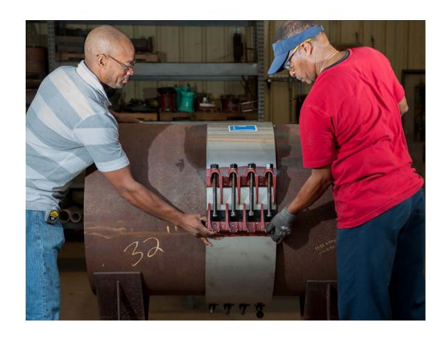
Bring other end of clamp to meet with the bolting lug section. Feed the bottom tapered gasket into place. Mesh top lug fingers and engage bolts.
