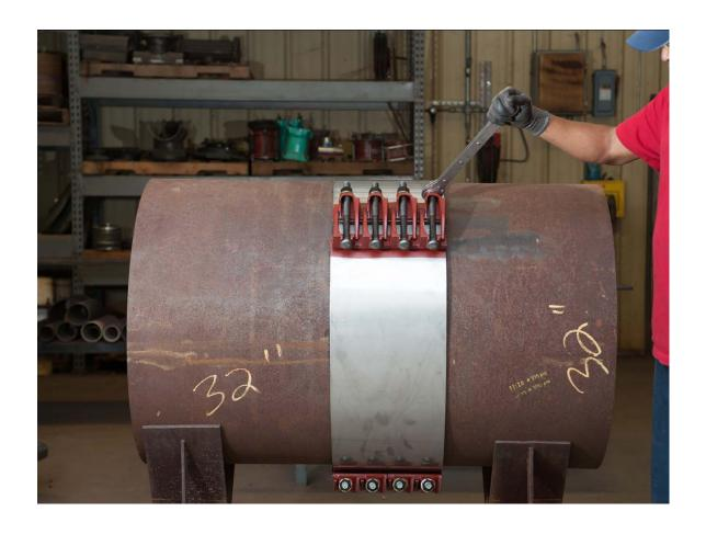
When oval neck bolts are engaged in the "ears" of the lug unit, proceed to tighten nut of each bolt on each clamp band section.
