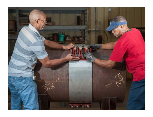
Loosely engage the bolts into the lug receiving ears and rotate the clamp in the direction of the arrow on the label (spraying pipe surface with soapy water will help this step). This aids in smoothing the tapered gasket edge and prevents leak channels caused by curled or folded gasket edges.
