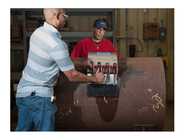
Position the clamp over the damaged area, check the visual mark to ensure close to center over the damage. Ensure the tapered gasket edge of each clamp section lies flat against the pipe.
