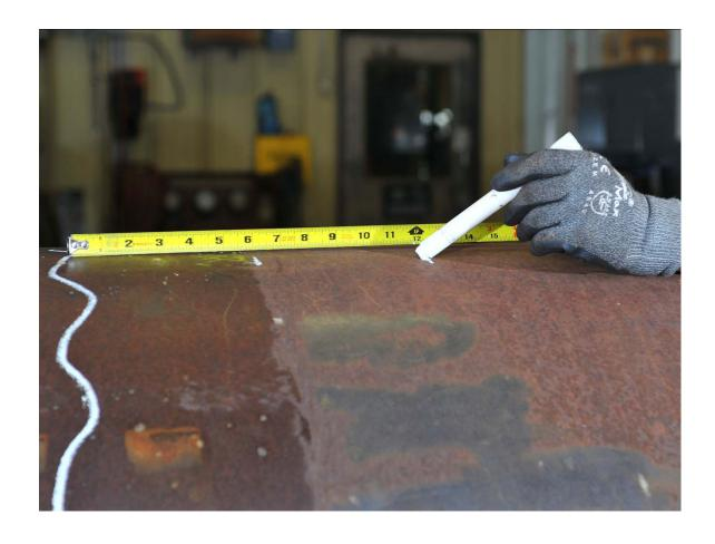
Trick of the trade: Using a tape measure and marking implement, place a mark on the pipe equal to width of the clamp. This presents a visual mark to center the repair clamp over the damaged area. (1/2 of this distance is centered)
