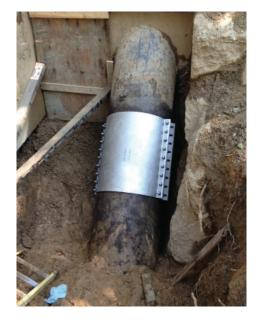
The JCM 6136 Heavy Duty Stainless Repair Clamp is available for all types and sizes of pipe. Options for this fitting includes: with or without threaded outlet; SBR, EPDM or Buna-N Gaskets. Call the JCM Inside Sales Team for product recommendations.
