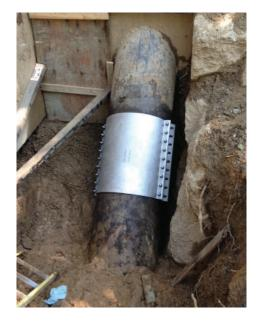
The JCM 136 Heavy Duty Stainless Repair Clamp is available for all types and sizes of pipe. Options for this fitting includes: 304 Stainless Steel, 316 Stainless Steel, SBR, EPDM or Buna-N Gaskets, 304 Stainless Hardware, 316 Stainless Hardware. Call the JCM Inside Sales Team for product recommendations.
