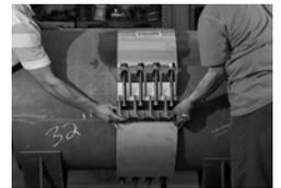
4. Tighten all bolts evenly to the following torque values, ensure torque values with calibrated field torque wrench:
