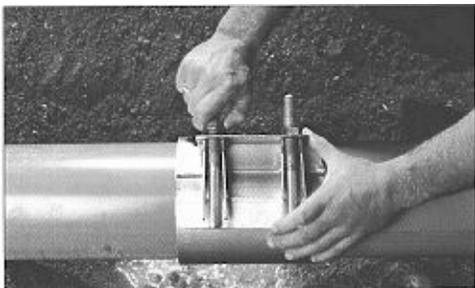
Complete tightening of the clamp by squeezing the lugs together and tighten the nuts to the appropriate torque levels.
