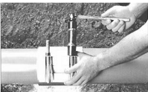
Tighten the nuts evenly with a hand wrench to the following torque values. *Trick of the Trade: Pneumatic wrenches could cause the stainless nuts to seize on the stainless steel studs.*
